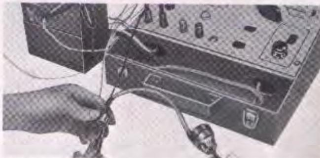
Fig. 6-80. Continuity test of the ignition switch
